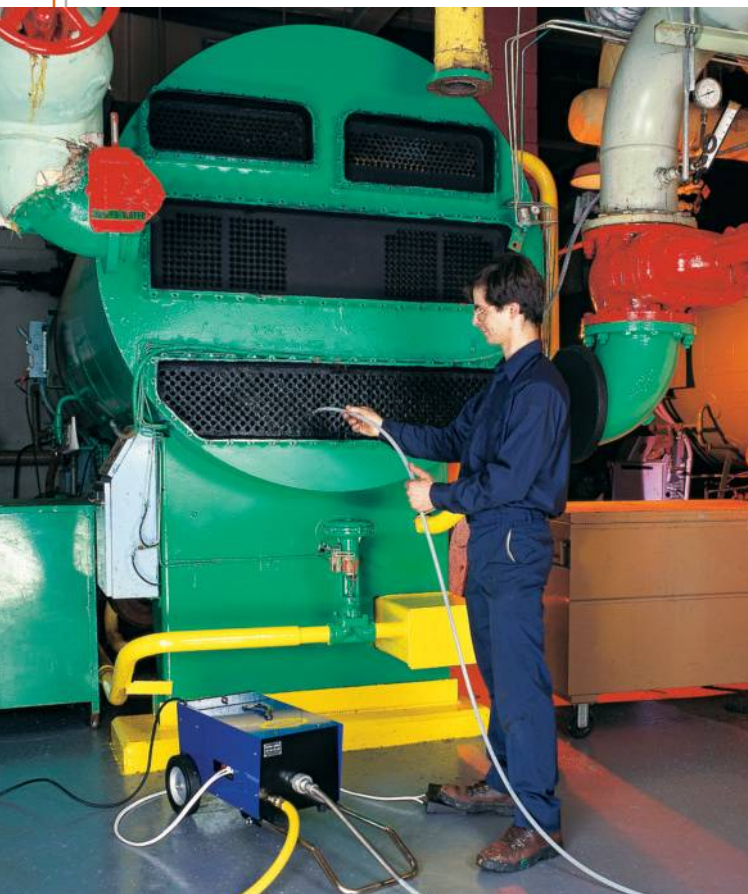
FIGURE 1 A REGULAR BOILER TUBE MAINTENANCE SCHEDULE CAN REDUCE FUEL CONSUMPTION BY 20% OR MORE.
