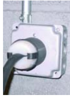
Insert twist lock plug
