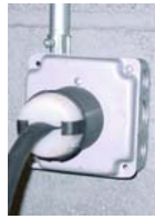
Insert twist lock plug
