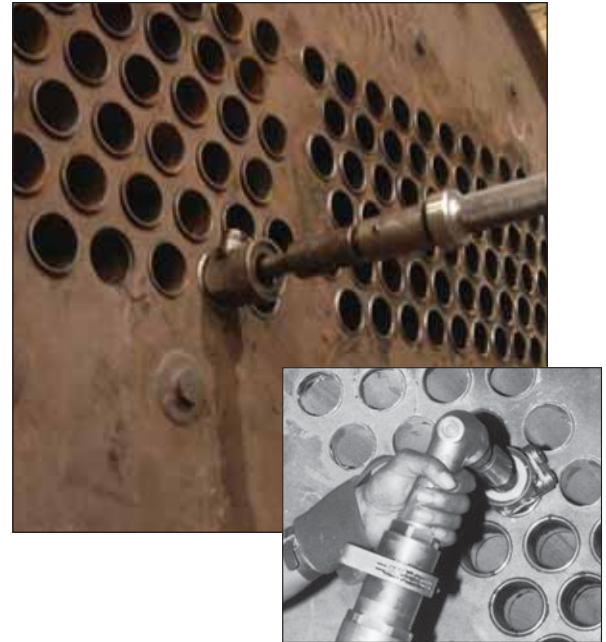
Combination Beading Expander in use with 909 Right Angle Pneumatic Tube Roller
