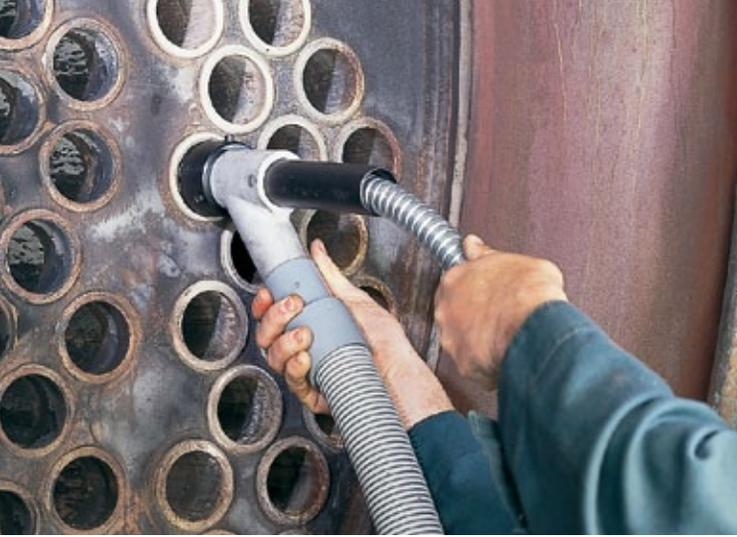
The Wils-Away™ 1000 Cleaning a Fire Tube Boiler
